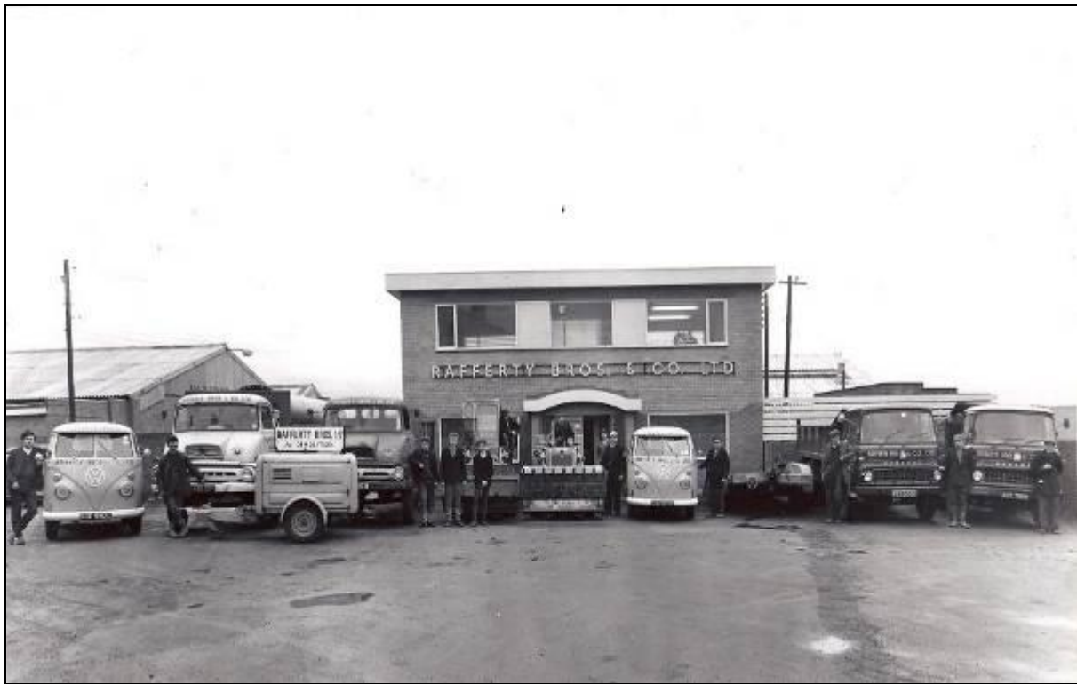
Development of Rafferty's Nash Peake Works and Plant in 1960's.
